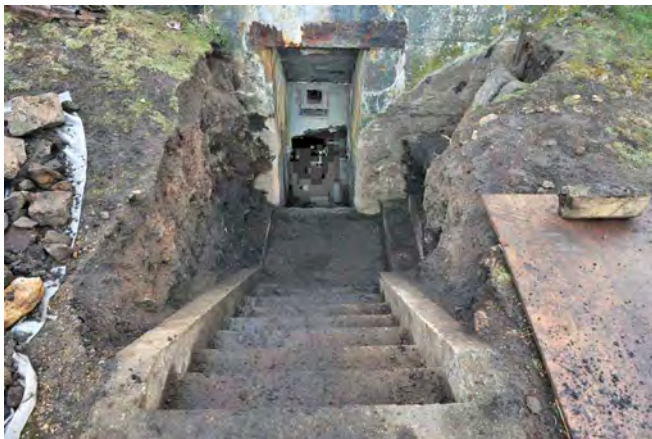
The recently excavated entrance to the FL232 bunker. Photo Tony Pike
